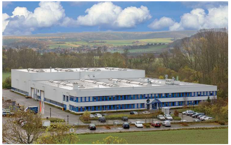
Kelvion Safety Heat Exchangers GmbH Firmensitz in Monzingen, Deutschland Kelvion Safety Heat Exchangers GmbH based in Monzingen, Germany
