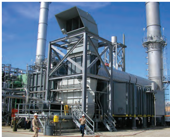
474,000 lb/hr 900 psig superheated boiler system.
