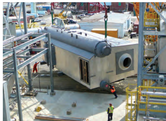
250,000 lb/hr 725 psig superheated boiler system.
